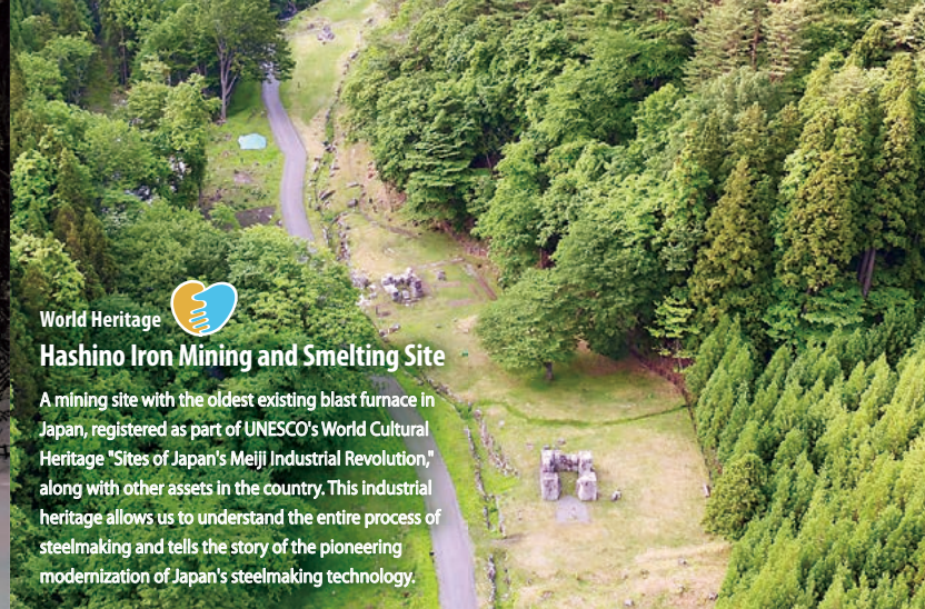
This location was chosen for the construction of blast furnaces due to the presence of iron ore as raw material, forests supplying wood charcoal as fuel, and rivers serving as the power source for waterwheels.
